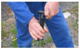
Step 8: Wind around the small drum at least three times to ensure contact and therefore conductivity with the exposed metal strip.
